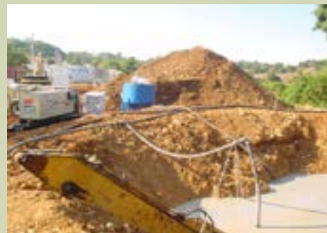
Slurry Wall Impermeable Construction
