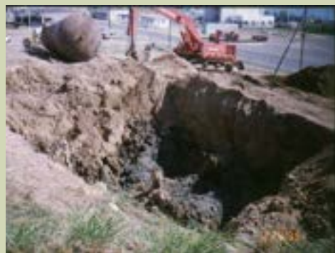
Underground Storage Tank Removal
