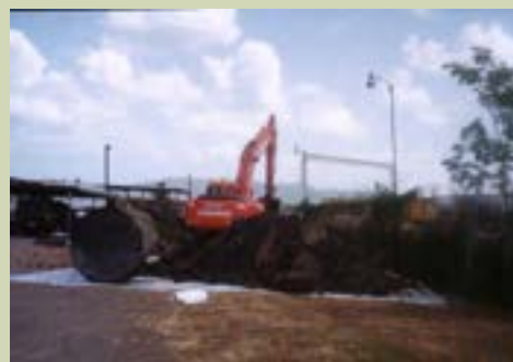
Underground Storage Tank Removal
