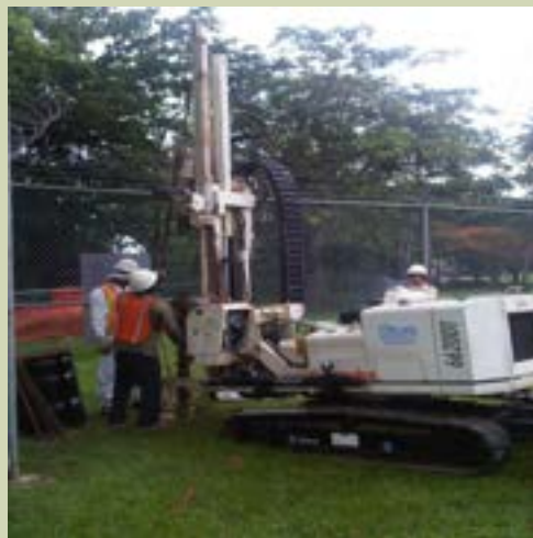
Soil & Groundwater DPT Sampling
