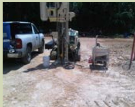
DPT Substrate Injection Project
