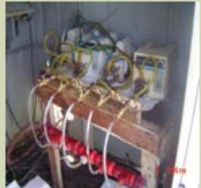
Product Recovery Pump System
