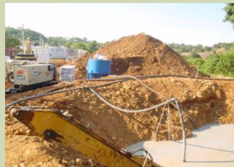
Slurry Wall Impermeable Construction
