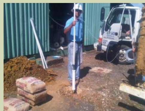
Perozone Injection Wells Project
