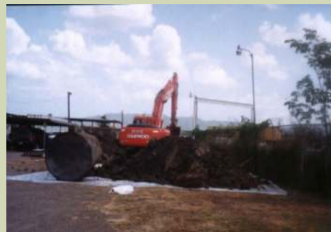
Underground Storage Tank Removal
