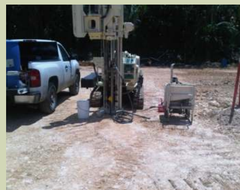
DPT Substrate Injection Project
