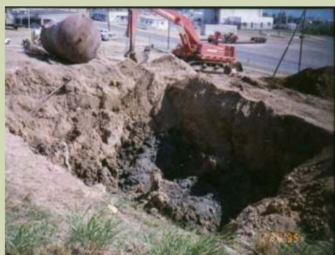
Underground Storage Tank Removal
