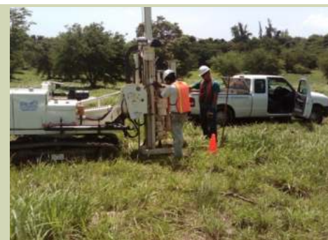
Site Investigation Project
