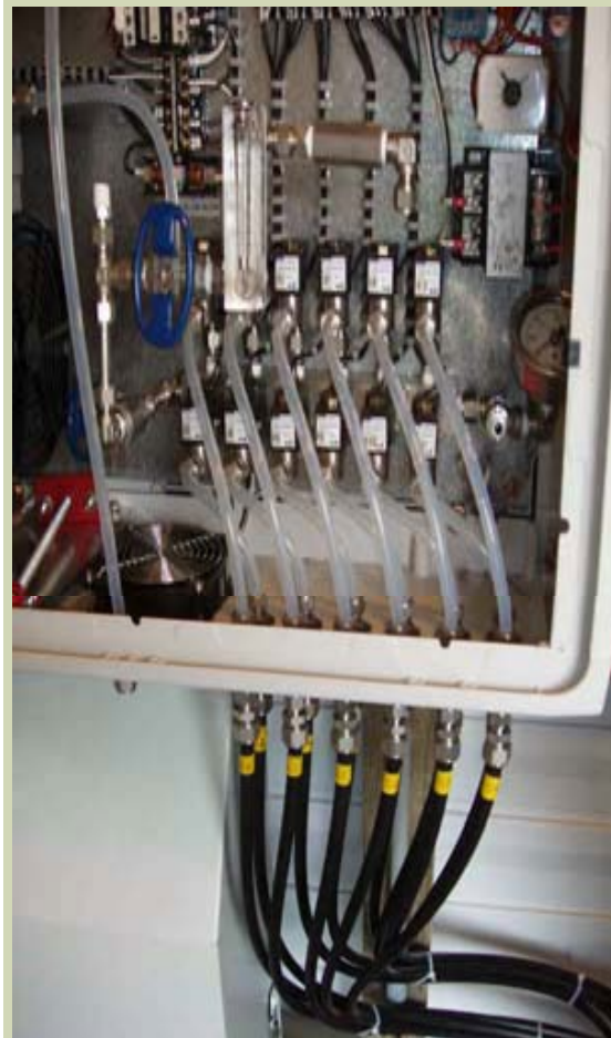
Perozone (Chem-Ox) Injection System
