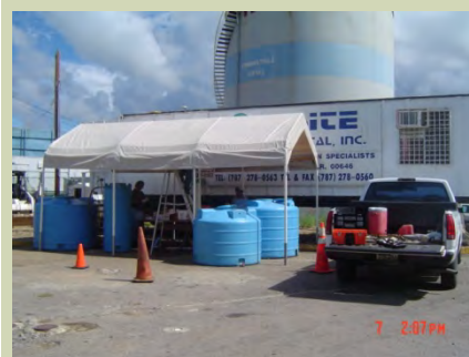
In-Situ Bio-Slurping System
