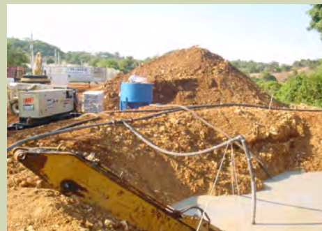
Slurry Wall Impermeable Construction
