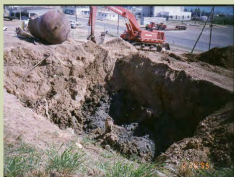
Underground Storage Tank Removal
