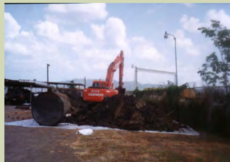
Underground Storage Tank Removal
