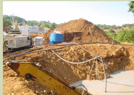
Slurry Wall Impermeable Construction
