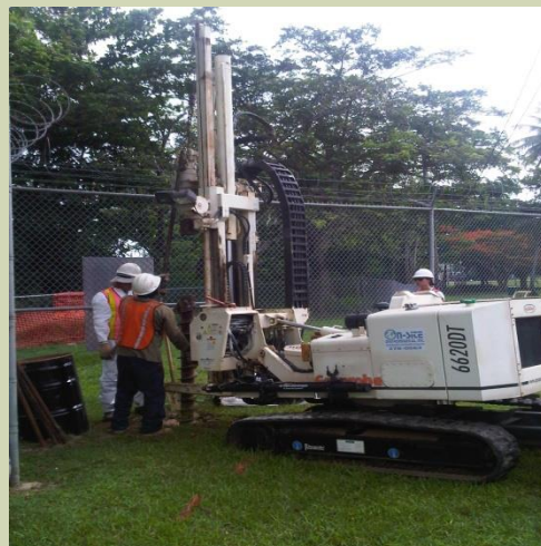
Soil & Groundwater DPT Sampling
