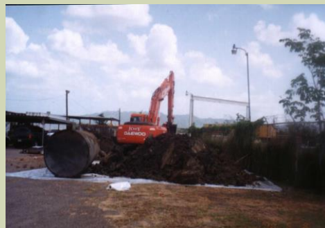
Underground Storage Tank Removal
