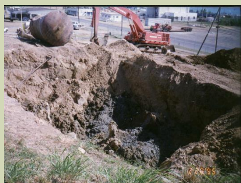
Underground Storage Tank Removal
