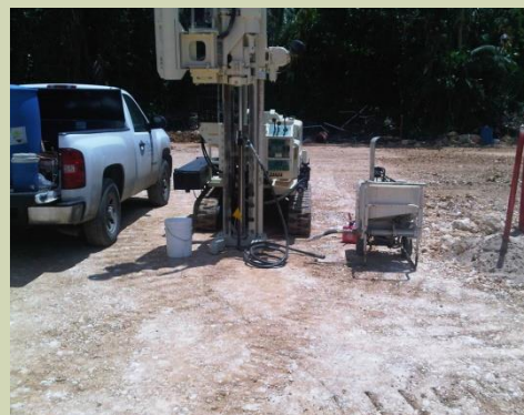
DPT Substrate Injection Project
