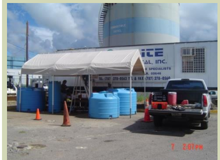
In-Situ Bio-Slurping System
