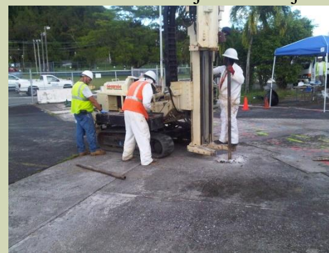
Free Product Recovery Project
