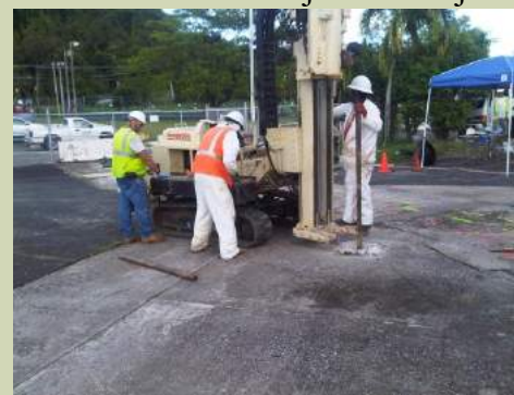
Free Product Recovery Project
