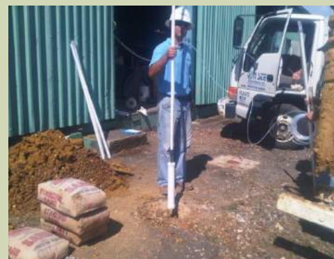
Perozone Injection Wells Project
