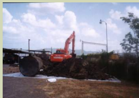
Underground Storage Tank Removal
