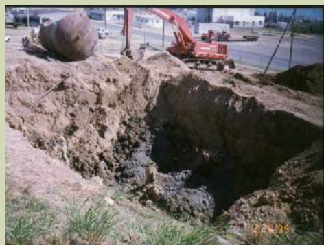
Underground Storage Tank Removal
