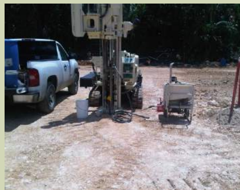
DPT Substrate Injection Project
