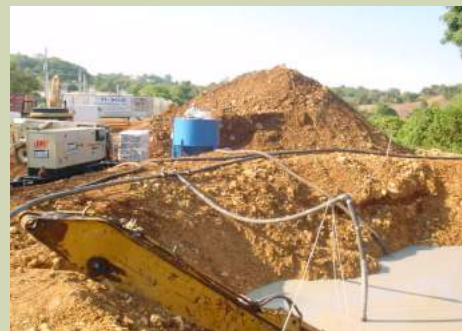
Slurry Wall Impermeable Construction
