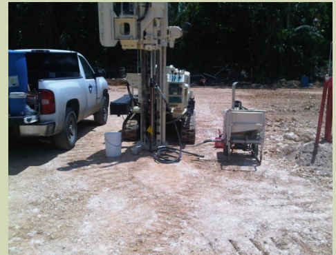
DPT Substrate Injection Project
