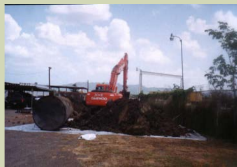
Underground Storage Tank Removal
