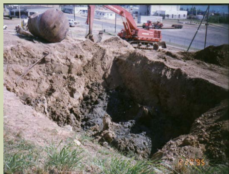
Underground Storage Tank Removal
