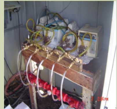
Product Recovery Pump System
