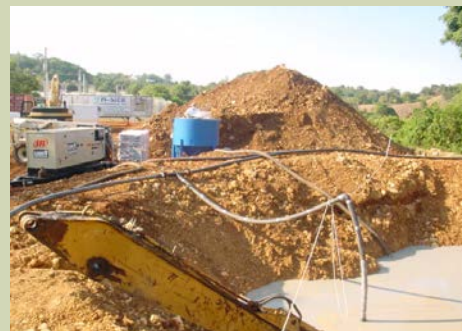
Slurry Wall Impermeable Construction
