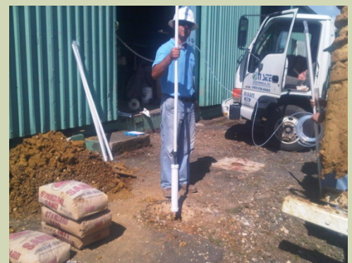
Perozone Injection Wells Project
