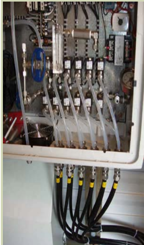
Perozone (Chem-Ox) Injection System
