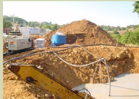
Slurry Wall Impermeable Construction
