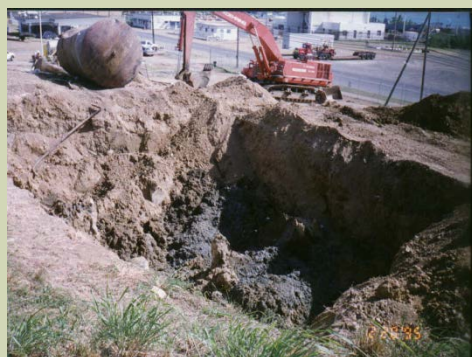
Underground Storage Tank Removal
