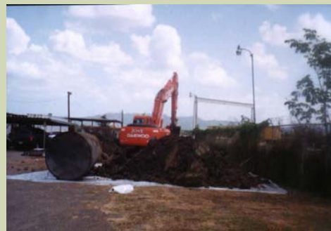
Underground Storage Tank Removal
