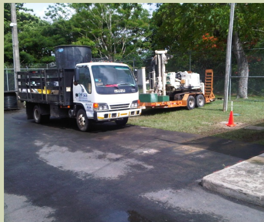
DPT/HSA Drilling Equipment
