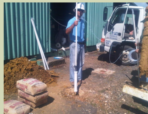
Perozone Injection Wells Project
