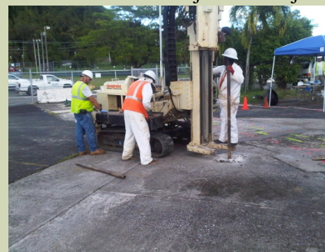
Free Product Recovery Project
