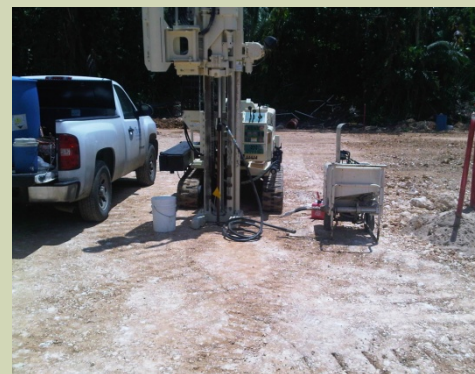
DPT Substrate Injection Project
