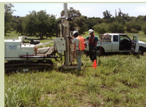
Site Investigation Project
